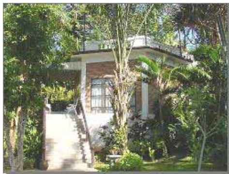
Villa Roof Top
